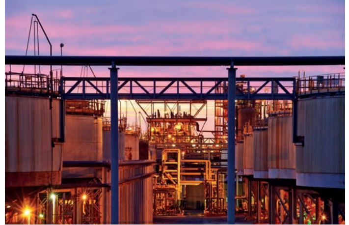
Fig 3. Alcoa operates this alumina refinery at Wagerup in Western Australia. (This photograph was provided courtesy of the Australian Aluminium Council.)
